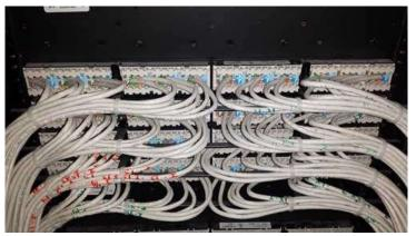
Note that strain-relief is to be used for all copper cabling. Cables will be dressed in to the strain-relief with either Velcro or zip ties. Further, all cable bundles will be dressed in at no greater than 36" segments where visible and no more than 60" segments where not in cable tray.
